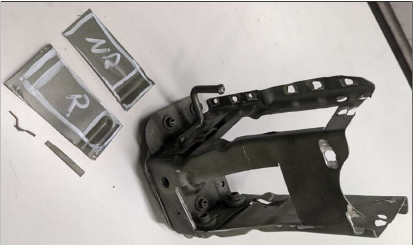
Image 5: This photograph shows the extracted samples cut from the chassis section, and marked 'R' (Repaired), and 'NR' (Not Repaired).
