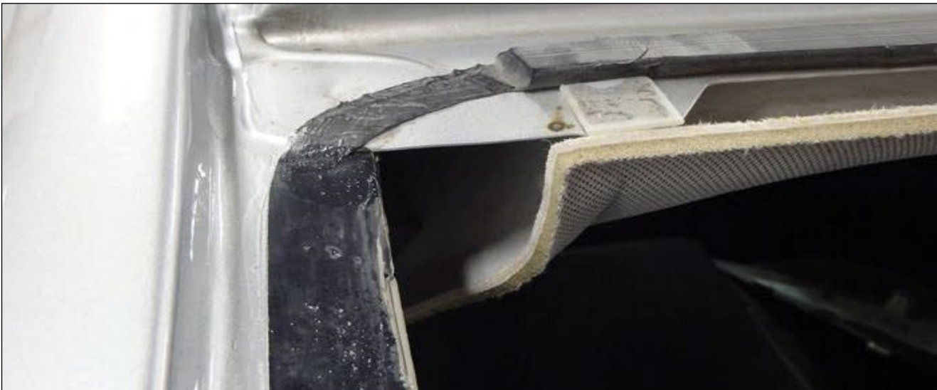
Image 7: Pinchweld flange Inspection and Preparation. Close-cut the original urethane down to a thickness of 1 mm - 2 mm. Clean with water and dry with a clean cloth.
