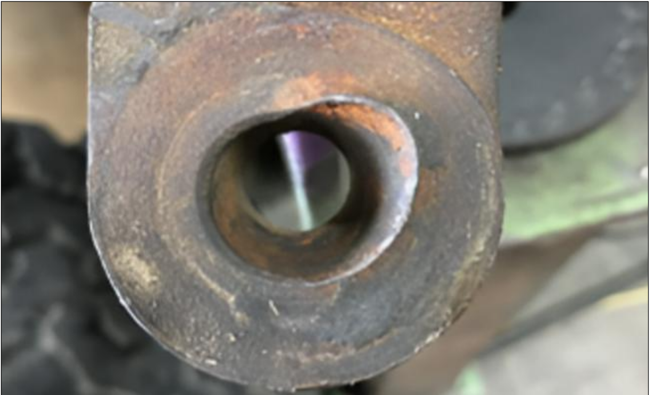
Image 22: The tapered hole on this steering knuckle has been distorted from an impact, breaking the taper lock between it, and the connecting tie rod ball joint.
