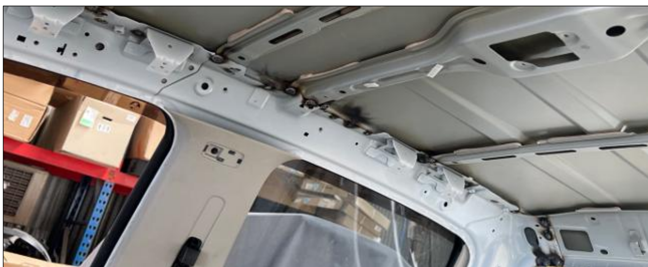
Images 15 and 16: Weld point detail – roof structure to existing inner cant rail and body-side structure.
