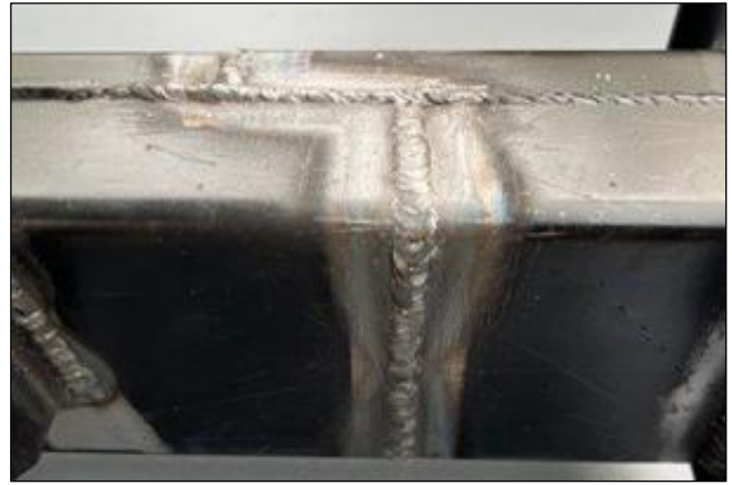
Image 8: Staggered cut sectioning joint
