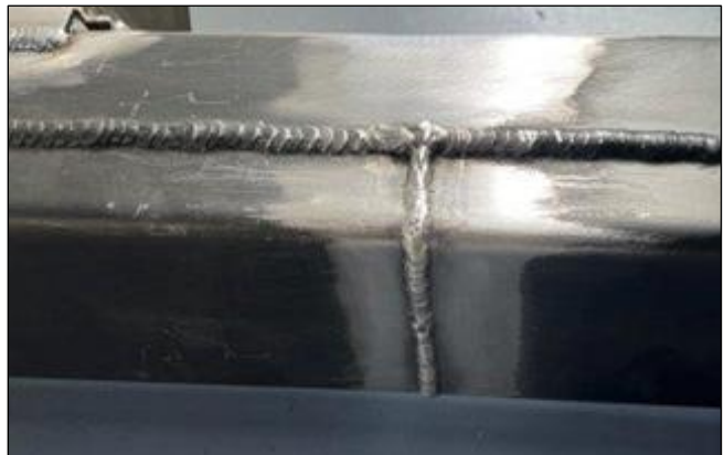
Images 32 and 33: The DPT procedure is completed only after the final surface condition of the weld has been achieved.
