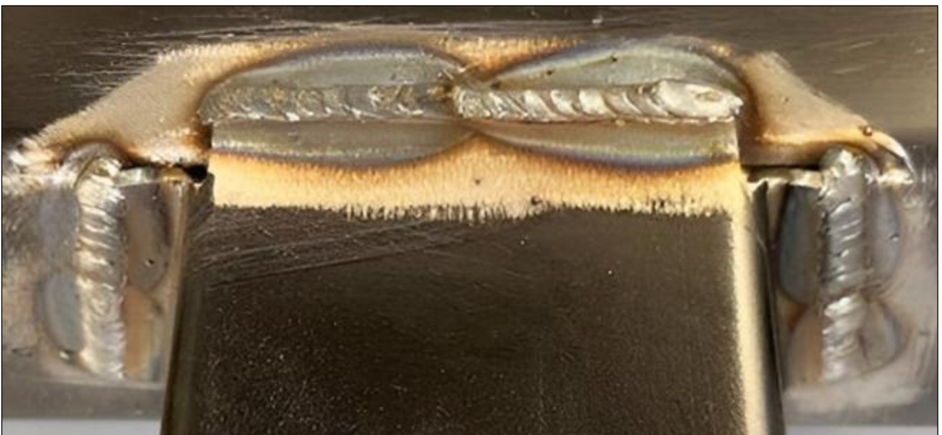
Image 29: Weld in quadrants, staggering the location of each weld run to control distortion and the HAZ.
